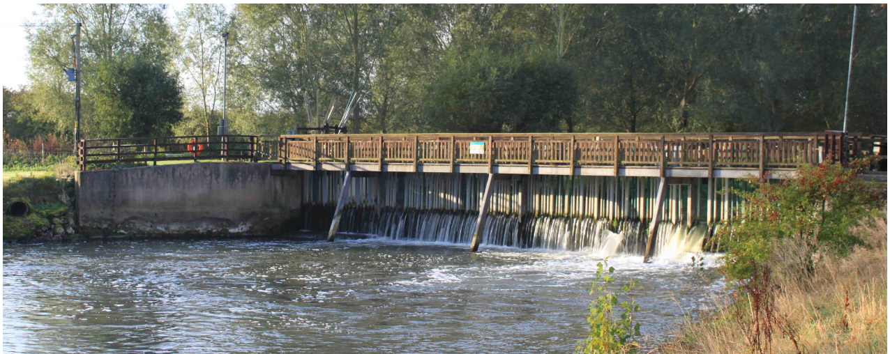
Refurbished Paddle and Rymer weir at Northmoor, October 2011
