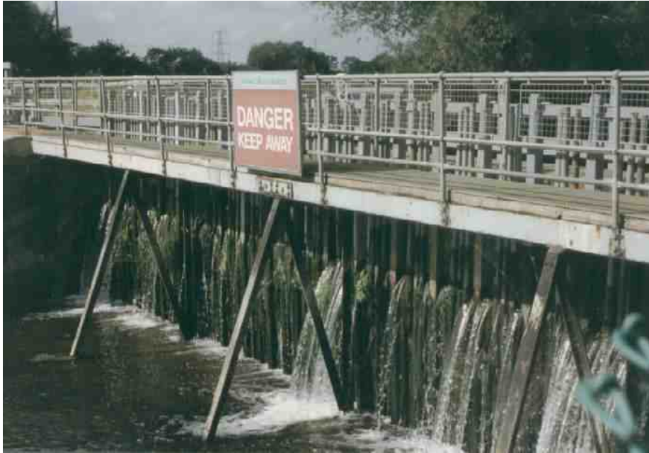
Northmoor Weir (sometime prior to the refurbishment work in 1995)
