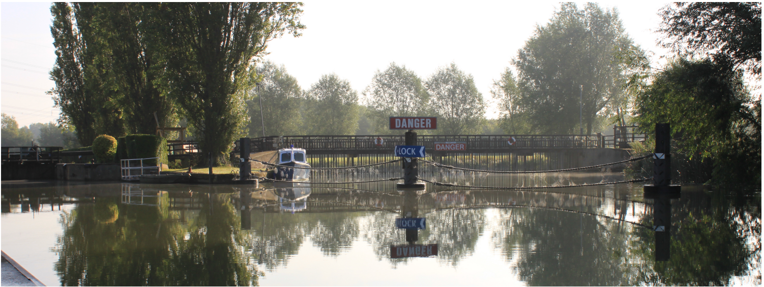
The lock and weir at Northmoor, one of only two weirs still operated using only Paddles and Rhymers
