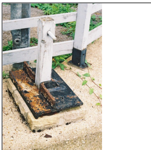
THA/MT/ E/3: Segment of weir sill (removed in 1995 to allow for fish) with cut down rymer, set on the weir side.
