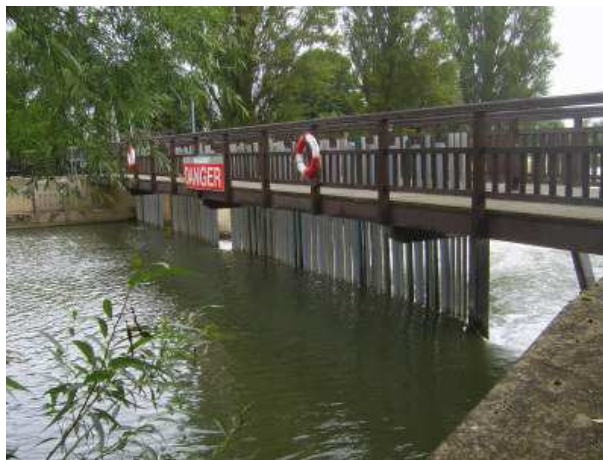
Upstream side of weir, from SSE on 19/08/2008 (THA/MT/SV107483)
